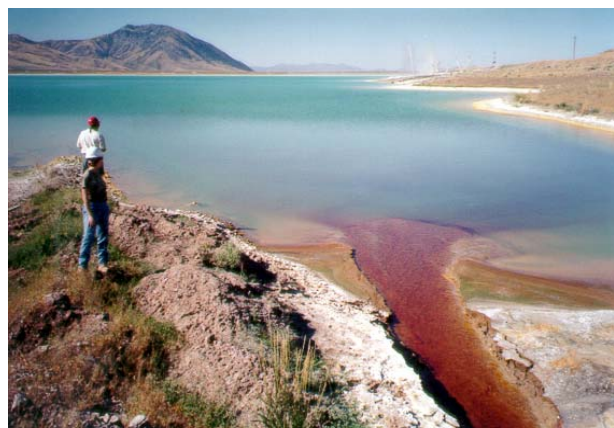
Acid and metalliferous drainage entering a tailings dam at a gold mine in western USA.
