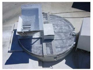
Below ground hydrated lime Figure 6. Thickener / clarifier tank. Figure 5. storage, mixing and dosing system.
