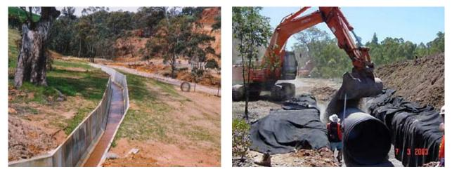
Figure 2. Dawesley Creek diversion drain. Laying pipe for the underground segments of the drain (right) and open channels (left).
