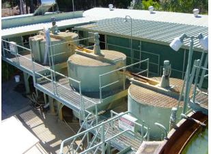
Acid drainage from the site is Figure 3. pumped to the North AMD holding pond (shown) prior to treatment.
