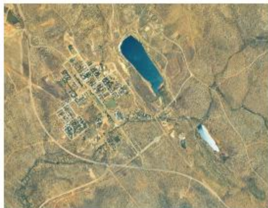
Fig. 3. Pine Creek Minesite in August 2000, showing completed rehabilitation works. Note the proximity of the flooded Enterprise Pit to the township of Pine Creek
